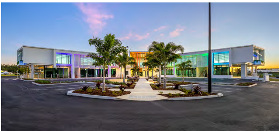
Compliance reached with Tactile Indicators installed on the kerb ramp at dusk
